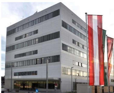
Headquarter RCPE GmbH – Graz, Austria © RCPE GmbH
