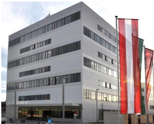
Headquarter RCPE GmbH – Graz, Austria © RCPE GmbH
